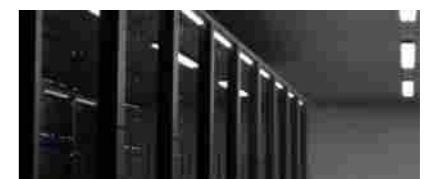
Data Center Management
